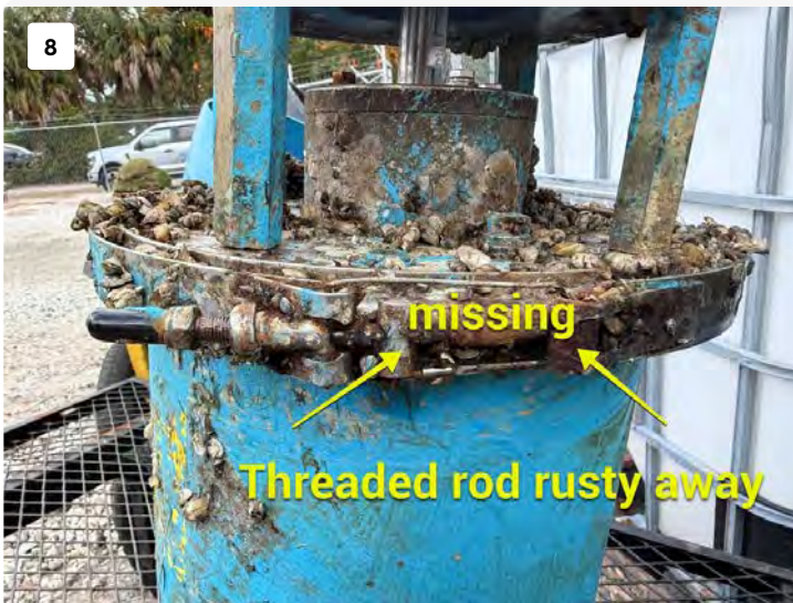
316 stainless steel components not being used by manufacturer.
